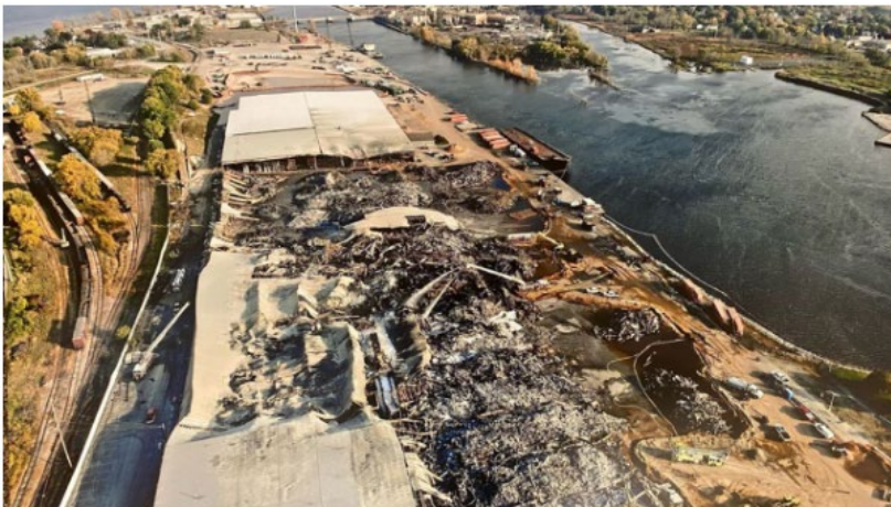
(Huge warehouse fire caused PFAS spike in Menominee, Marinette water - mlive.com)
